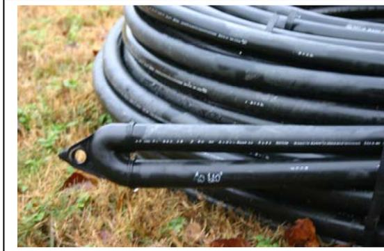
The U-bend of high density polyethylene pipe is a prefabricated and factory pressure tested heat fusion, which will be placed at the bottom of a 270-foot-deep borehole. This roll of pipe will fill one of 172 boreholes at SME's headquarters facilities and will carry a 55-year warranty.
